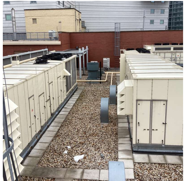
Roof 1 - West View
