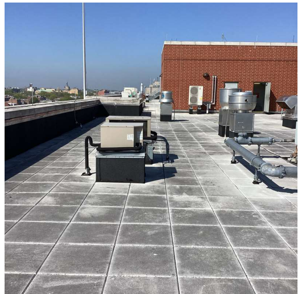
Roof 1 - Southwest View
