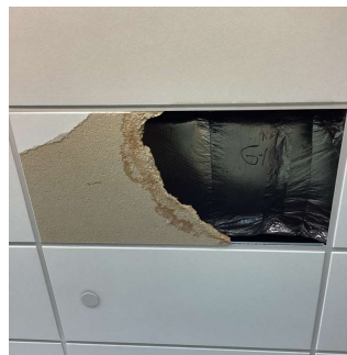
Roof 1 - Room 508 (Roof 1 - Room 506, Gymnasium similar)
