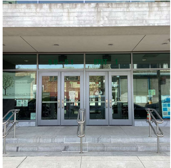
Facade A - 98th Street
