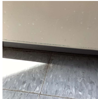
Facade F - Corridor near Stair C/2
