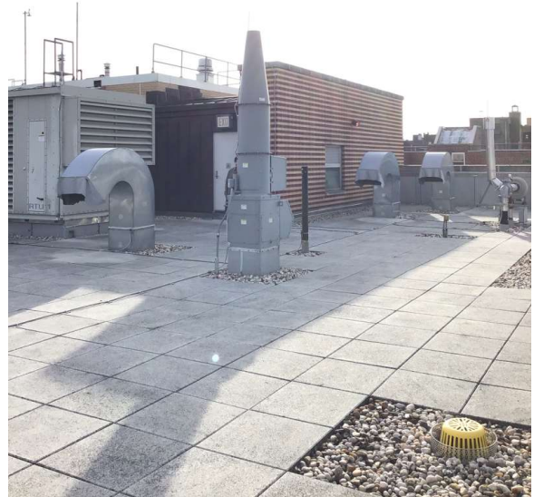
Roof 1 - Southeast View
