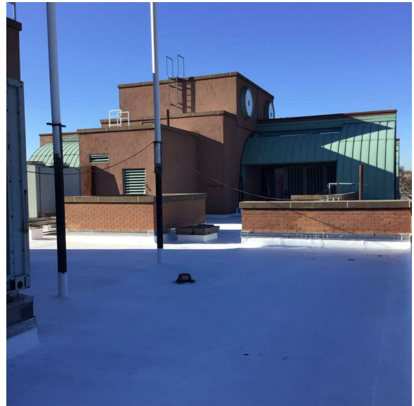
Roof 1 - Southwest View
