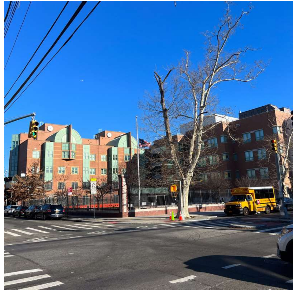
Corner of 99th Street and 34th Avenue - Northeast View
