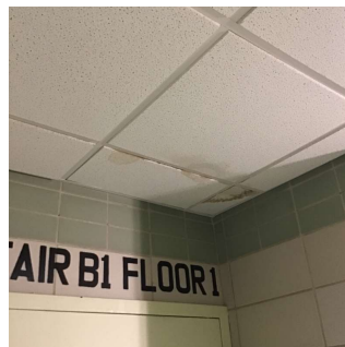
Corridor near Stair B/1
