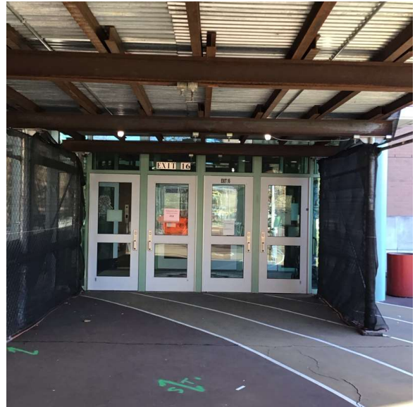
Facade A - 99th Street
