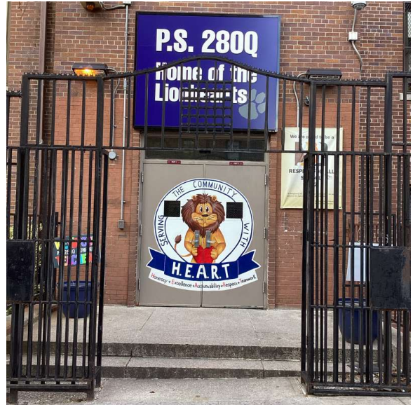
Facade A - 94th Street
