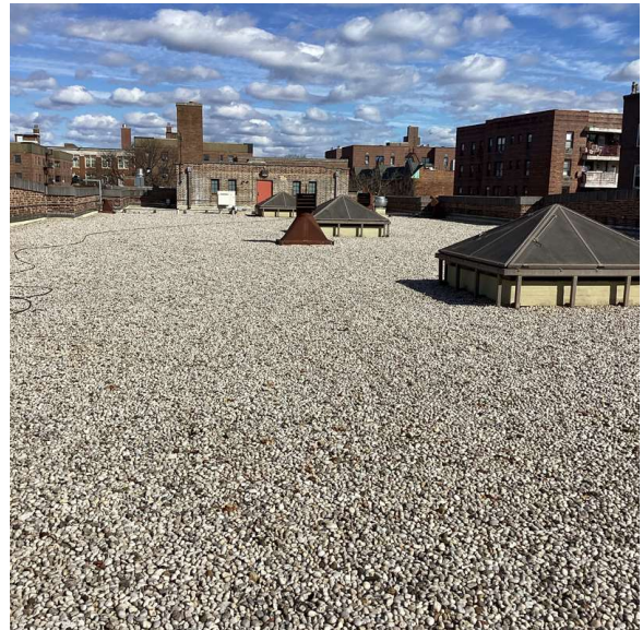
Roof 1 - Northwest View
