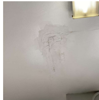
Facade B - Corridor near Stair A/2 (Old Building)
