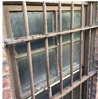
Facade H - Boiler Room
