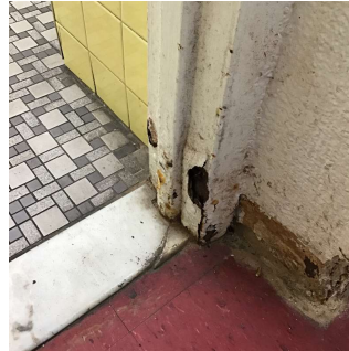
Basement - Boys OBrien Hall
