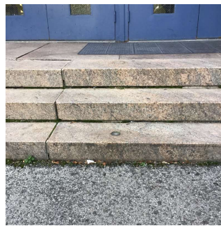
Facade A No violations recorded.
