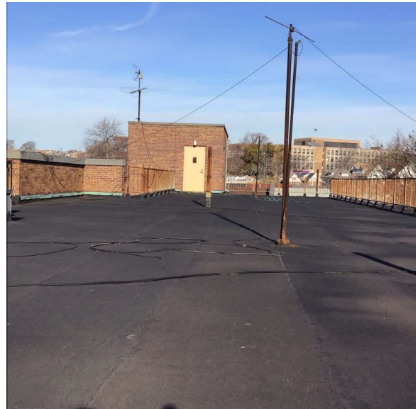
Roof 1 - Northwest View
