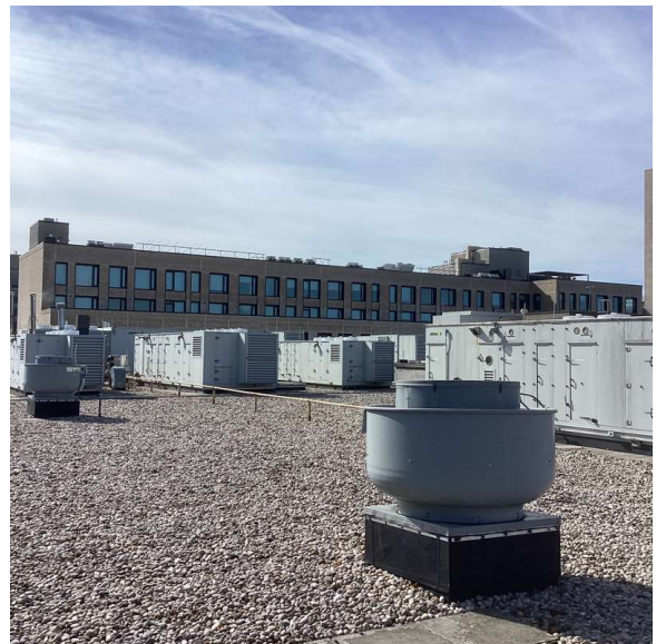
Roof 1 - Southwest view
