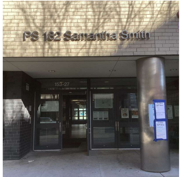
Facade A - 88th Street
