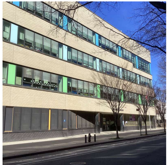
88th Street - Northeast view
