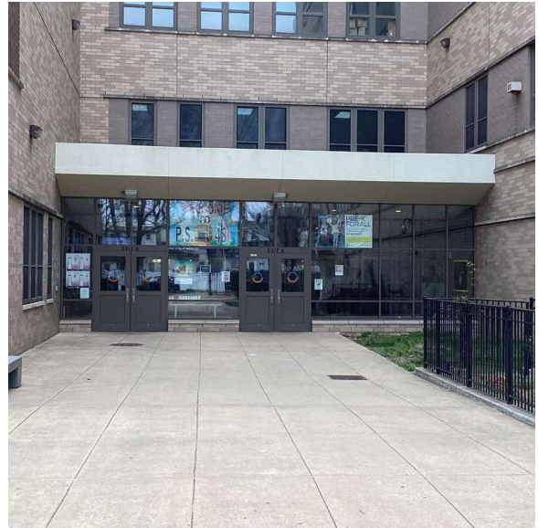
Facade A - 155th Street
