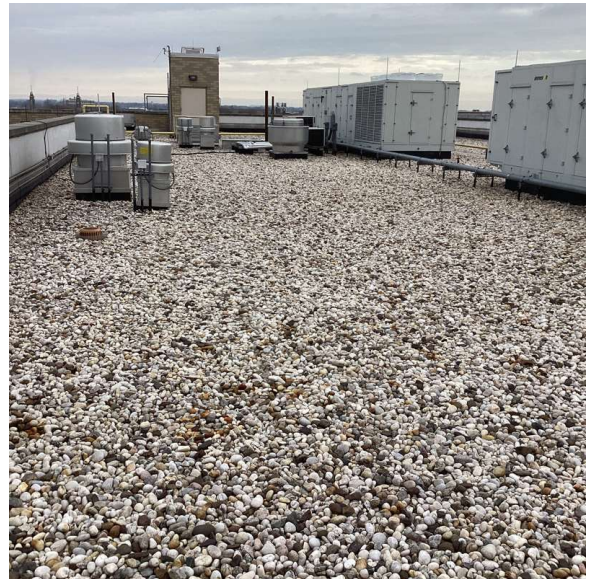
Roof 1 - East View
