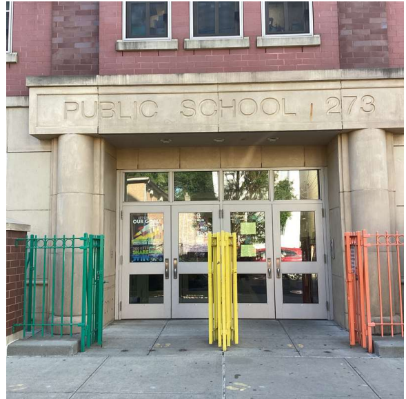
Facade A - 102nd Street
