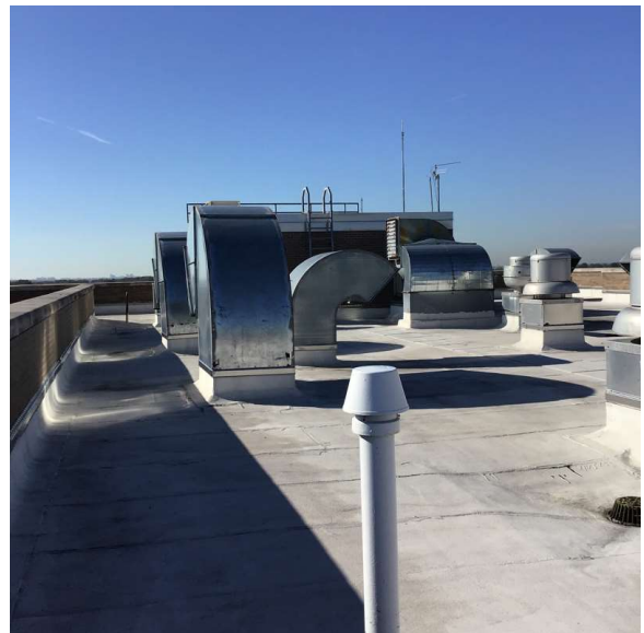
Roof 1 - Southwest view
