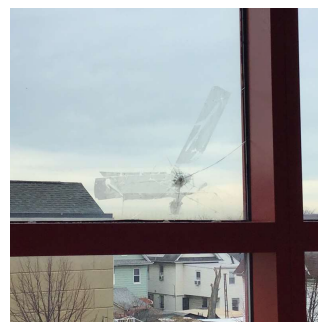
Facade C - Stair B/2-3 (Facade A - Stair A/3-4)
