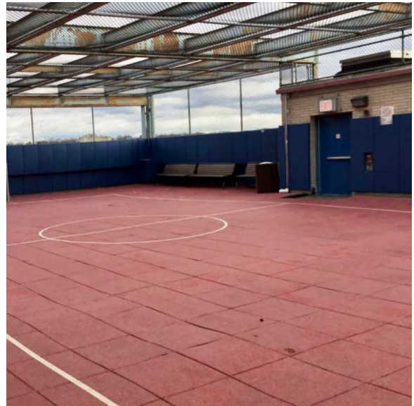
Roof 1 - Northeast View
