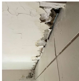
BH2 - Stair C
