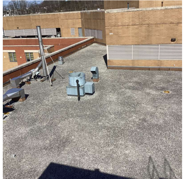
Roof 1 - Northwest view
