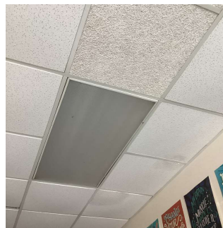
Roof 8 - Room 311, Stair C/3
