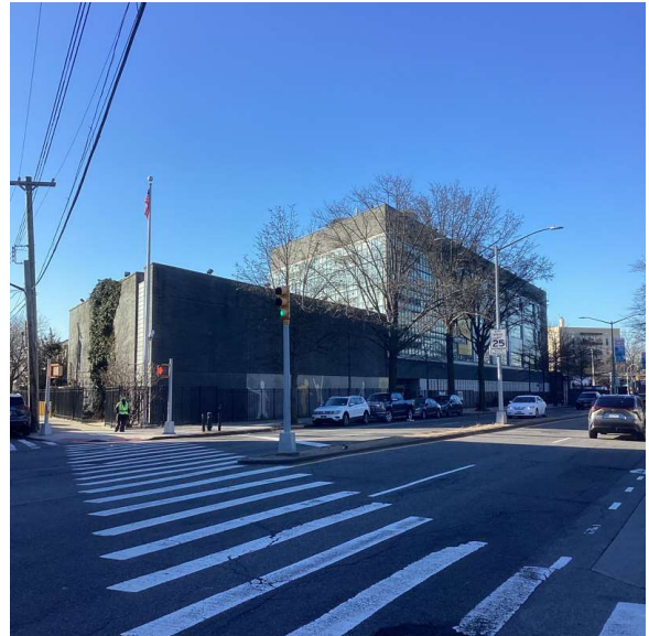
Corner of 224Th Street and Jamaica Avenue - South view
