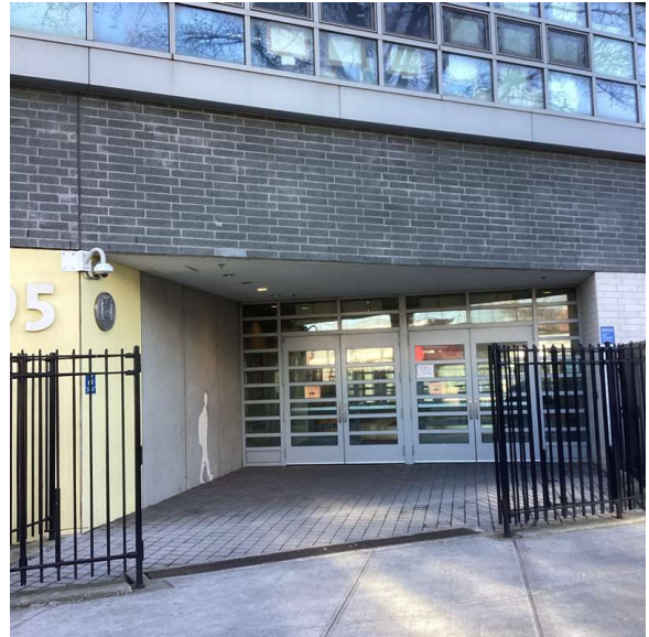
Facade A - Jamaica Avenue
