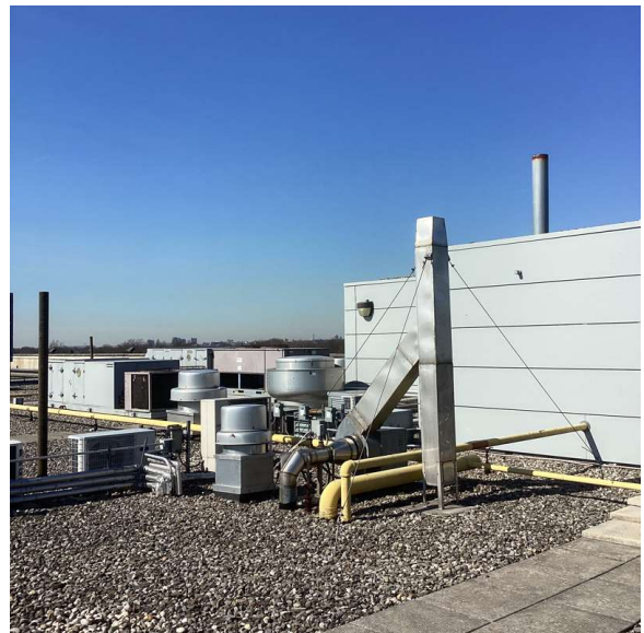
Roof 1 - West view
