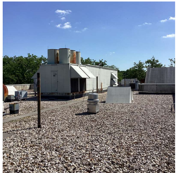
Roof 1 - Northeast view
