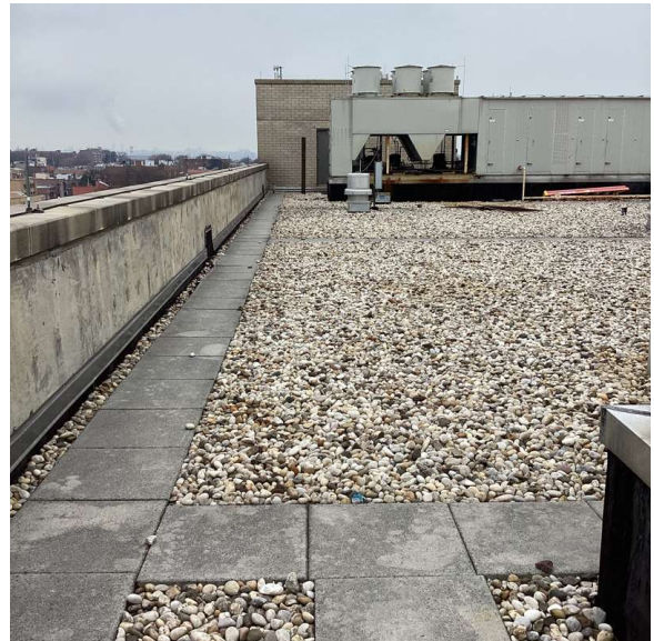
Roof 1 - Northwest View
