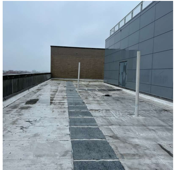
Roof 1 - Southeast View
