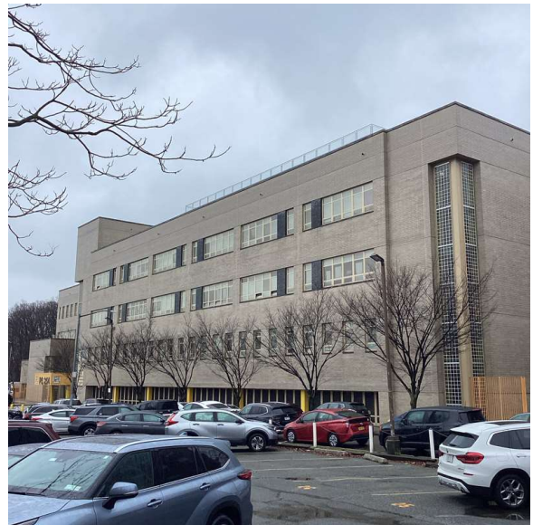
101st Street - South View
