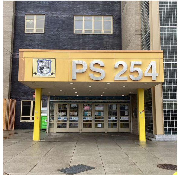
Facade A - 101st Street
