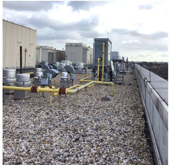
Roof 1 - East View
