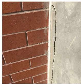
Facade E No violations recorded.
