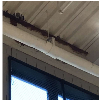
Roof 2 - Gymnasium No violations recorded.
