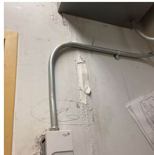
Roof 1 - Room 307 No violations recorded.
