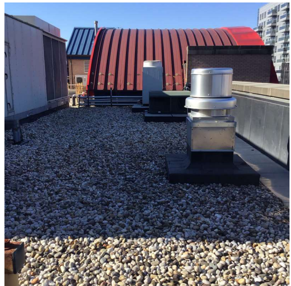
Roof 1 - Southwest View
