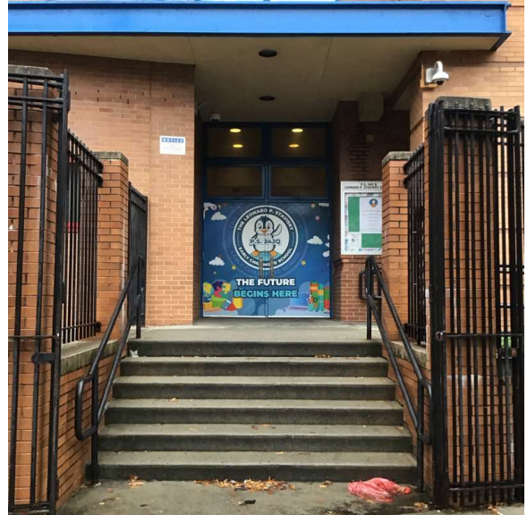
Facade A - 137th Street
