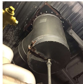
Roof 1 - Boiler Room, Fan Room
