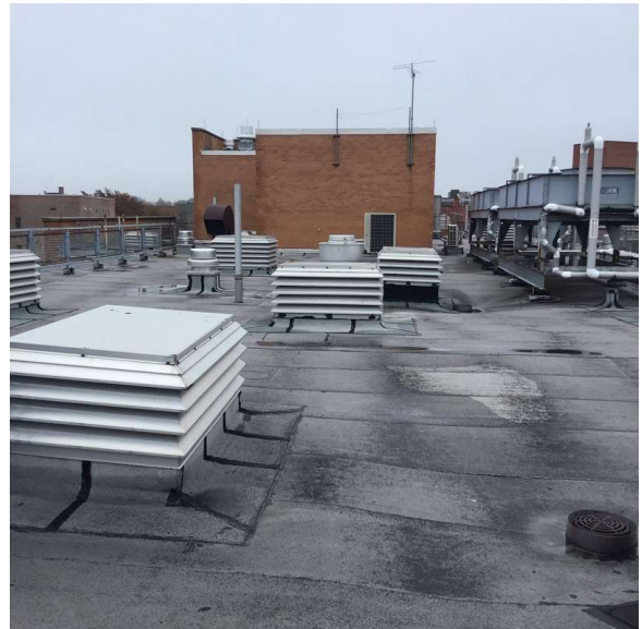
Roof 1 - Northeast View
