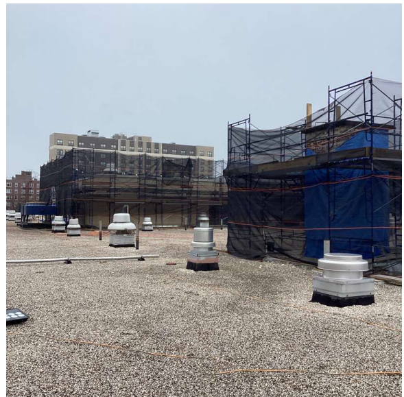
Roof 1 - North view
