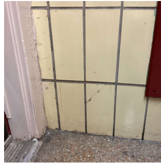
Stair C/Ground Floor - Vestibule
