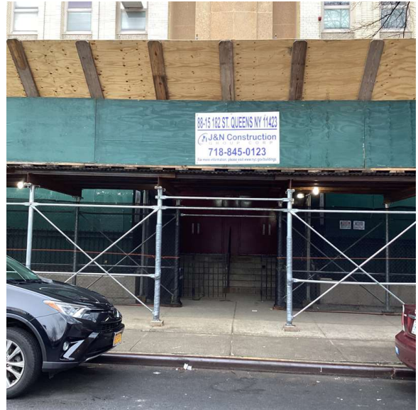
Facade A - 182nd Street
