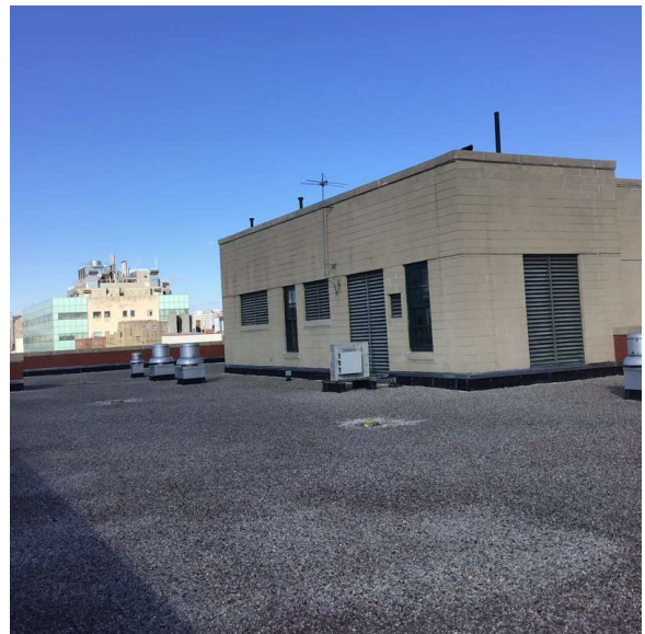
Roof 1 - South View
