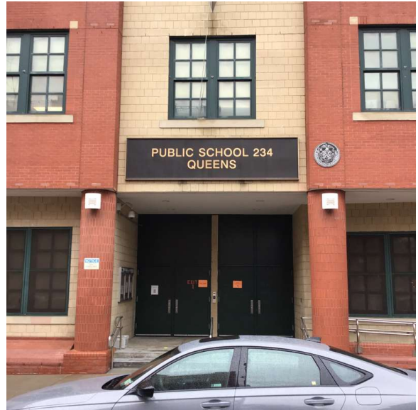
Facade A - 29th Street
