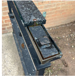
Facade A - Exit 2
