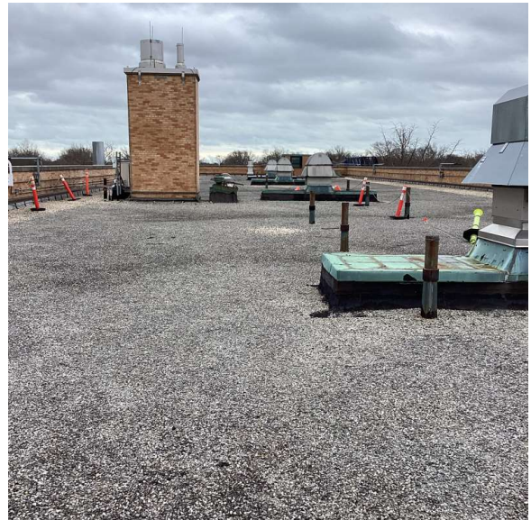
Roof 1 - Southeast View
