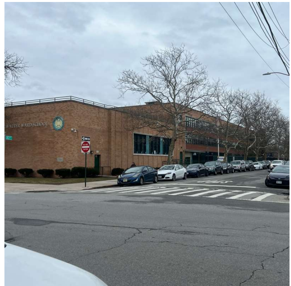
Corner of 153rd Avenue and 83rd Street - Southeast view
