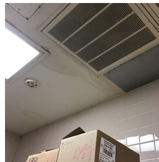
Facade B - Kitchen Dry Storage Room 108
