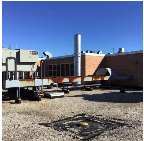
Roof 1 - Northeast view
