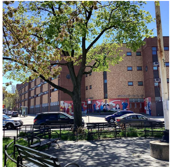
Corner of Junction Boulevard and 32nd Avenue - Southwest View
