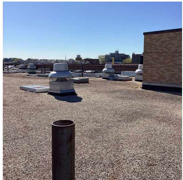
Roof 1 - Southeast View
