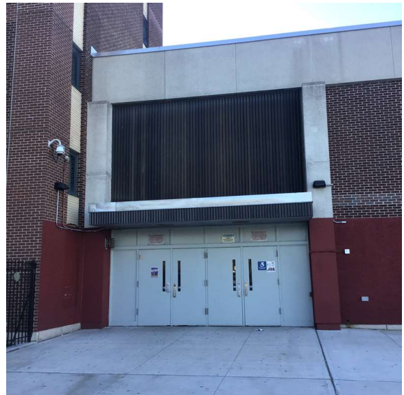
Facade A - Rockaway Boulevard
