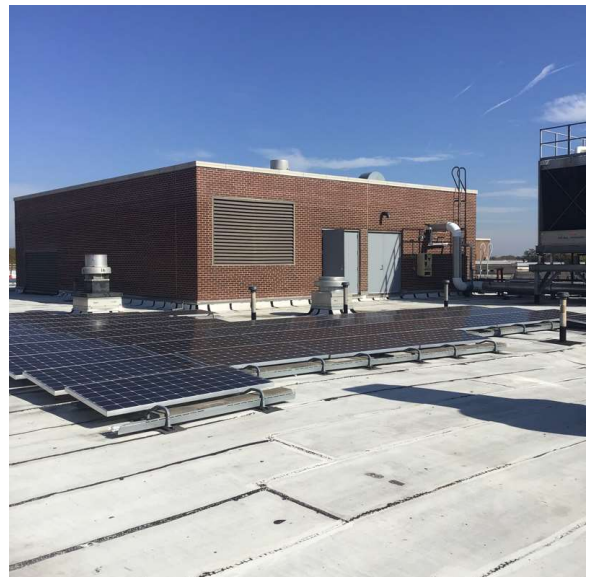
Roof 1 - Northeast view
