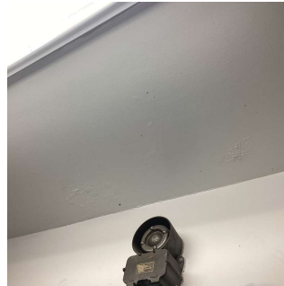
Corridor near Room 187
