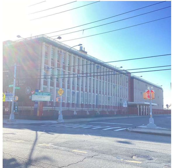
Corner of Rockaway Beach Boulevard and Beach 110th Street - Southeast view
