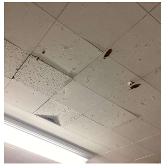
Corridor near Room 301
