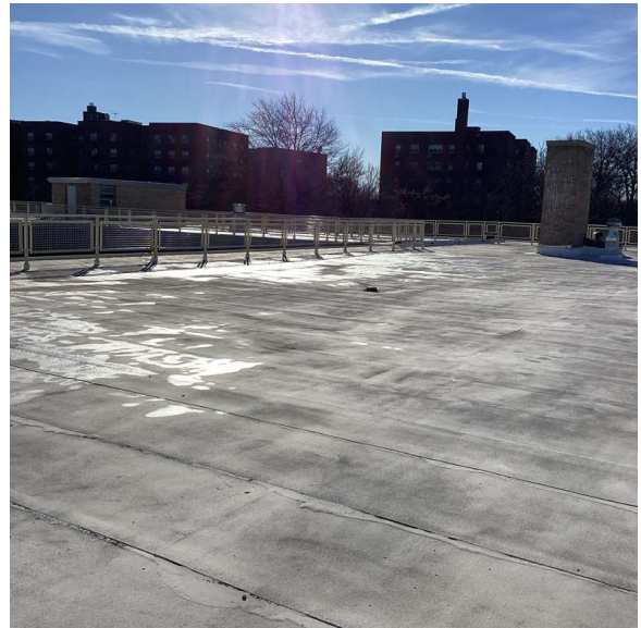
Roof 1 - Southeast View
