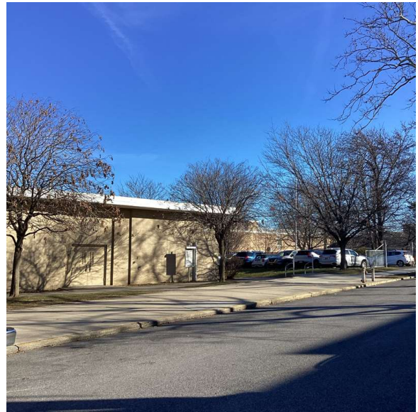
Gravett Road - Northeast View
