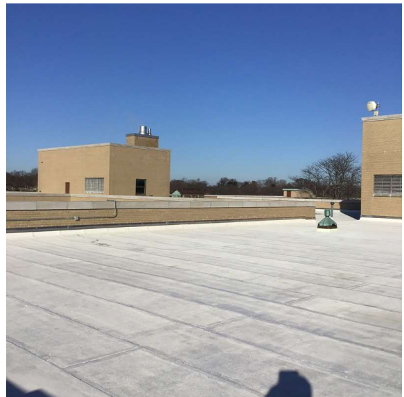
Roof 1 - Northwest view
