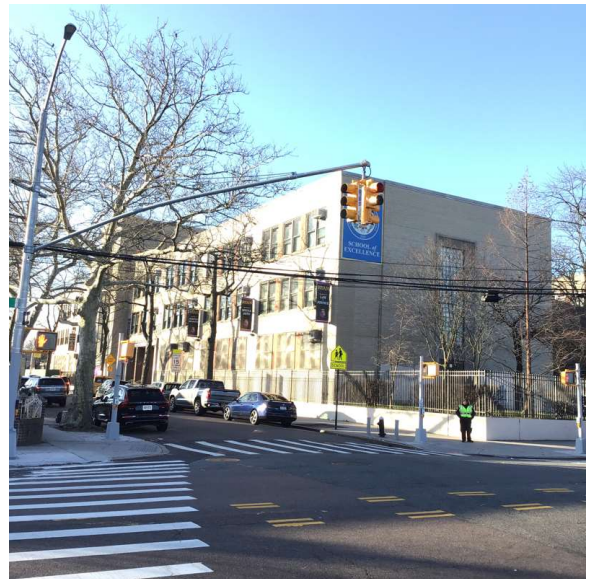
Corner of 175th Street and 64th Avenue - Southwest view
