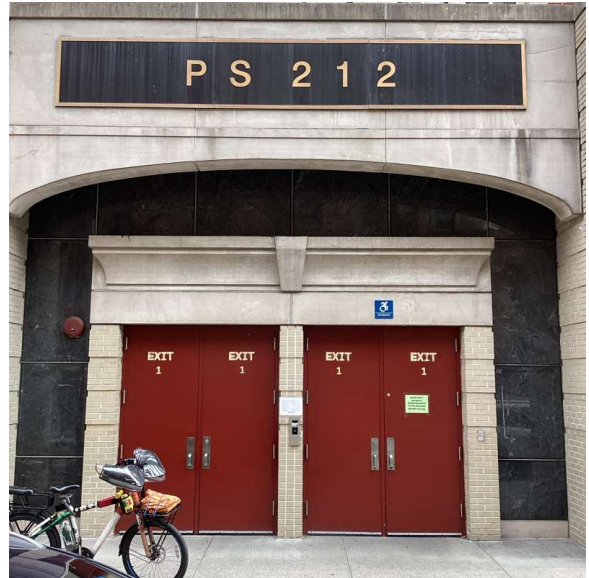
Facade A - 82nd Street
