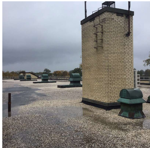
Roof 1 - Northwest View
