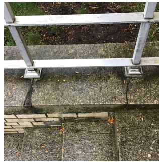
Facade G - Entrance 5 and 6
