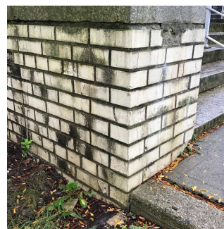
Facade G - Entrance 5 and 6
