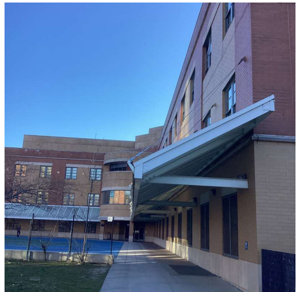
Facade A - East view
