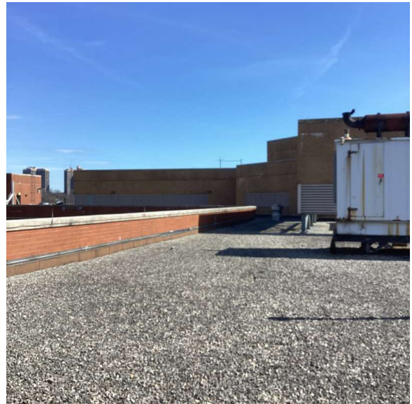
Roof 1 - Northeast view
