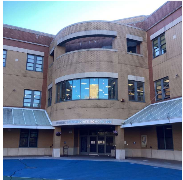
Facade A - East view
