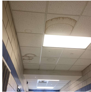
Corridor near Room 301
