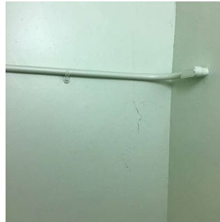
Stair Near Exit 8
