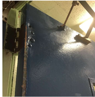
Entrance Right Side
