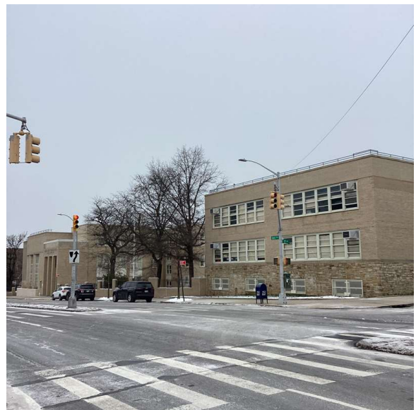
Corner of Bell Boulevard and 77th Avenue - North View
