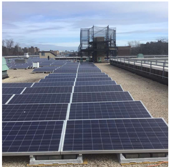
Roof 1 - Northeast View
