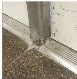
Facade A - Main Entrance No violations recorded.
