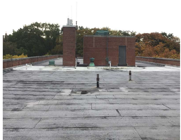
Roof 1 - South View
