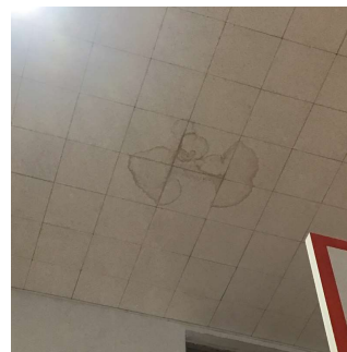
Roof 4 - Gymnasium (shown), Roof 1 - Stair DE/3
