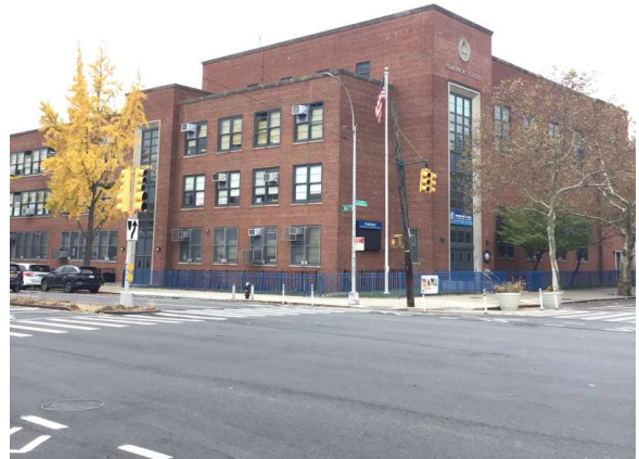
Corner of Jewel Avenue and 164th Street - Southwest View
