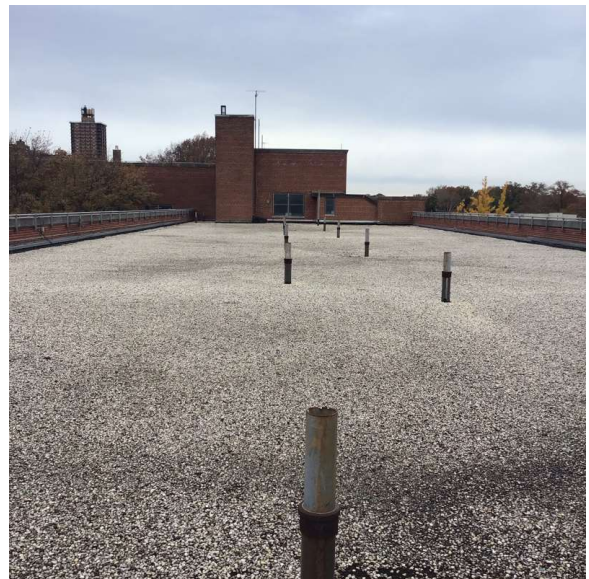
Roof 1 - North View
