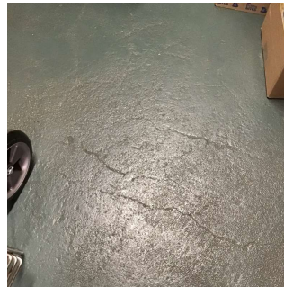
Storage Room Near Kitchen
