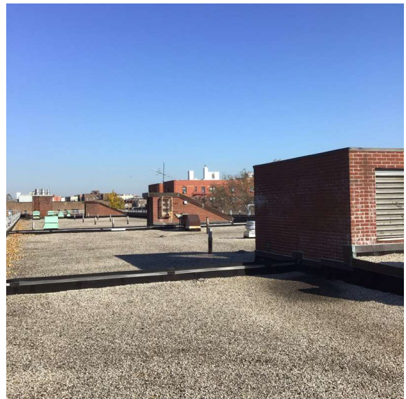
Roof 1 - South View
