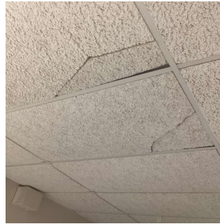
Corridor near Room 427
