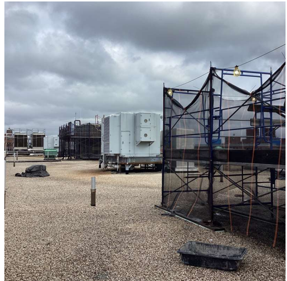
Roof 1 - Northeast view
