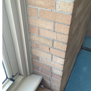
Corridor near Room B19 No violations recorded.
