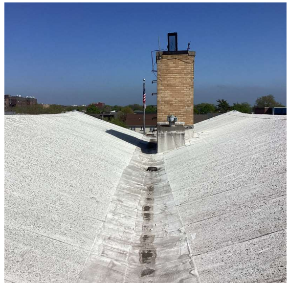
Roof 1 - East view
