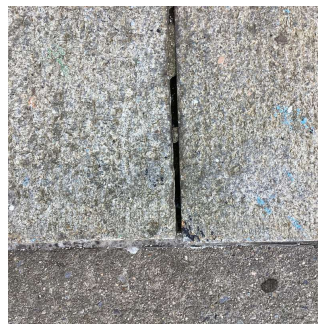
Facade H No violations recorded.
