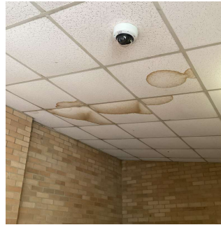
Corridor near Room 130
