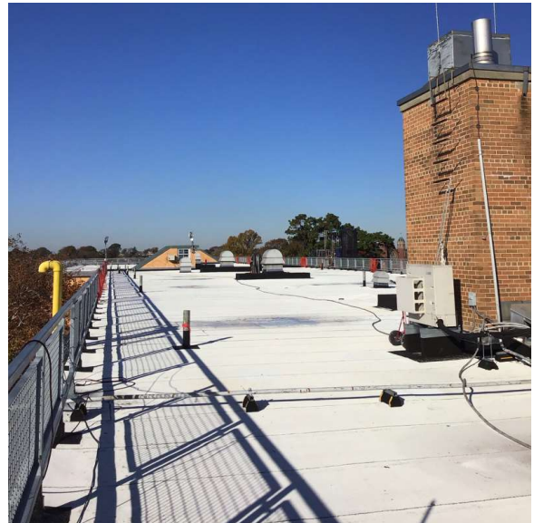
Roof 1 - Northwest View
