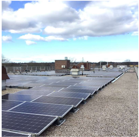
Roof 1 - North view
