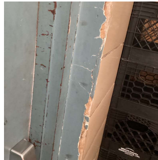
Near Exit to outside
