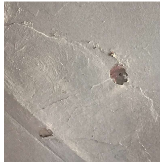
Facade A No violations recorded.
