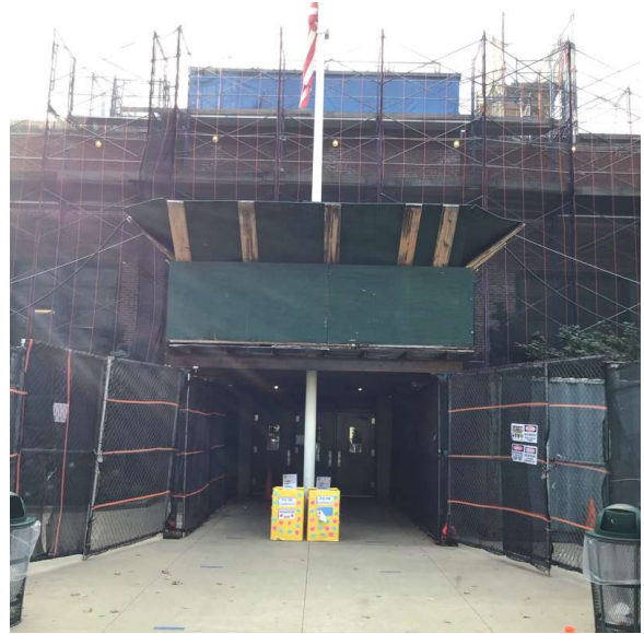
Facade A - 72nd Avenue
