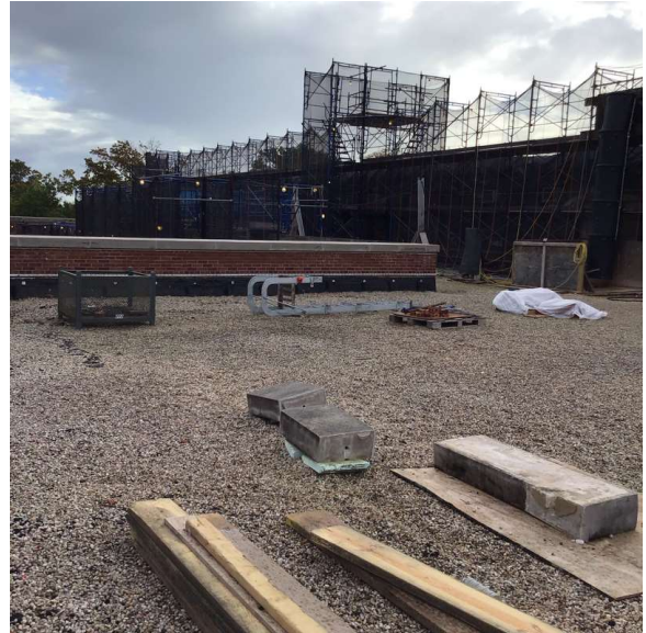
Roof 2 - Southeast View
