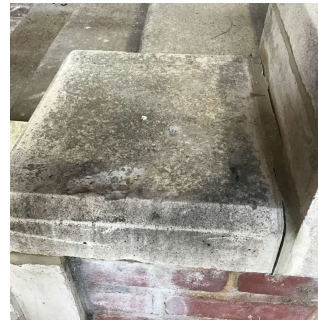
Facade D - Exit 3
