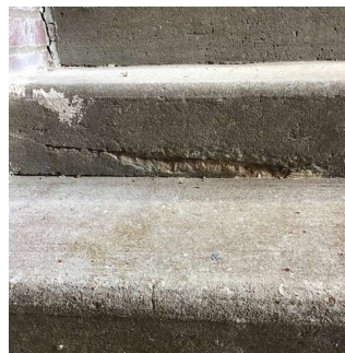
Facade D - Exit 3
