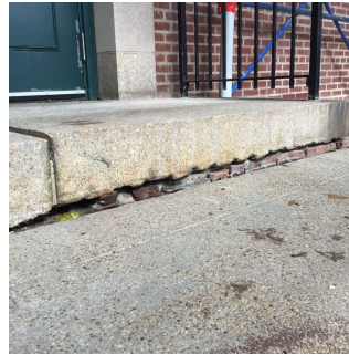
Facade C - Exit 4
