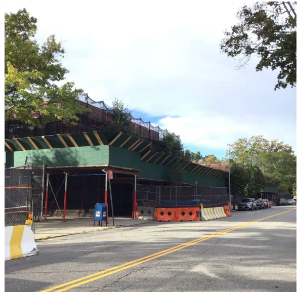
72nd Avenue - Southwest View
