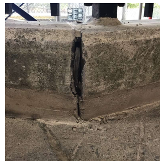
Facade D - Exit 3
