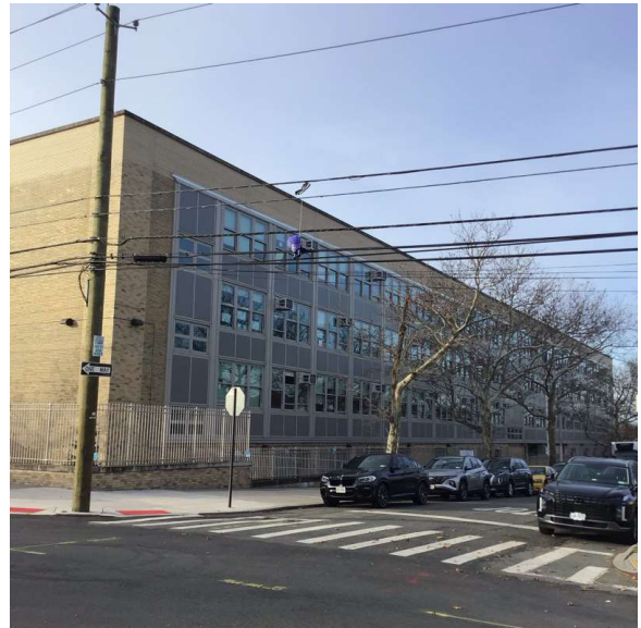
Corner of 149th Street and 25th Drive - Southwest View
