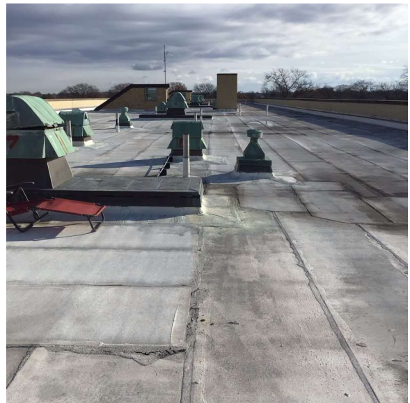
Roof 1 - East View
