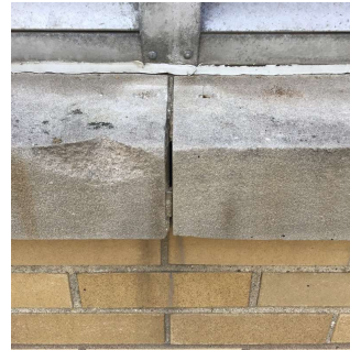
Facade E - Gymnasium Fan Room
