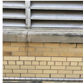
Facade E - Gymnasium Fan Room
