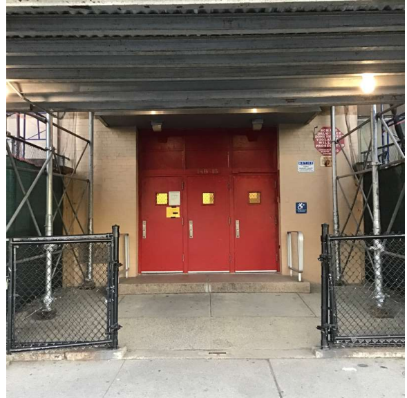
Facade A - 230th Street
