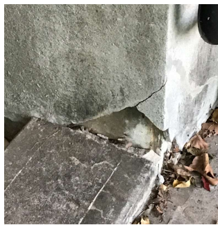
Facade B No violations recorded.
