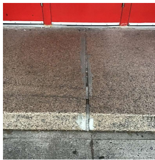
Facade A No violations recorded.
