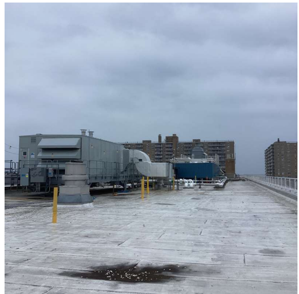
Roof 1 - South view
