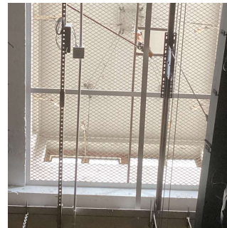
Roof 4 - Auditorium Stage
