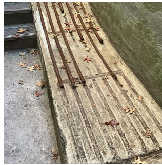
Facade C - AW4
