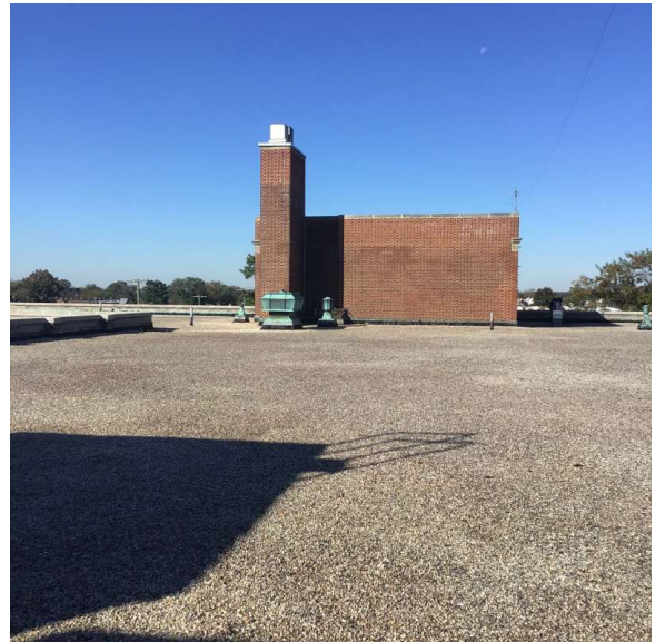
Roof 1 - West view
