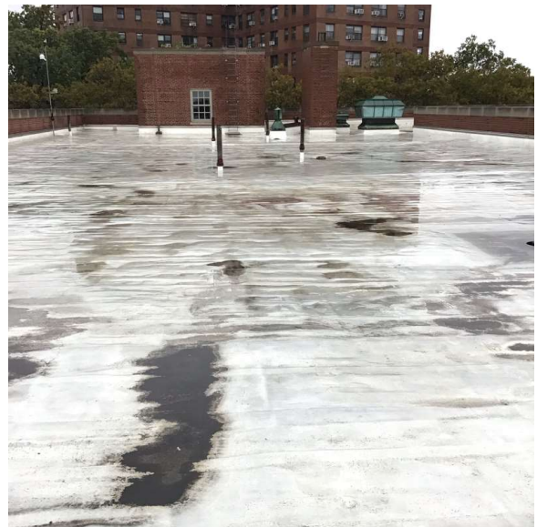
Roof 1 - Southwest View
