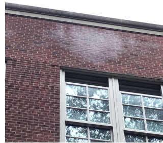
Roof 1 - Facade B
