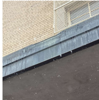
Facade H - Exit 5
