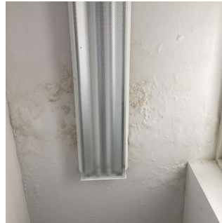
BH3 (Stair F)
