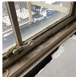
Facade H - Stair A-B/2 (similar throughout Auditorium, Gymnasium, Stair A-B)
