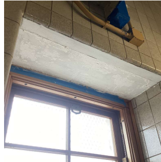
Facade G - Stair EF/3 (Facade F - Room 212, Facade E - Stair CD/3, similar throughout)
