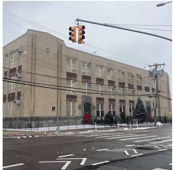
Corner of 53rd Avenue and 202nd Street - Southwest View
