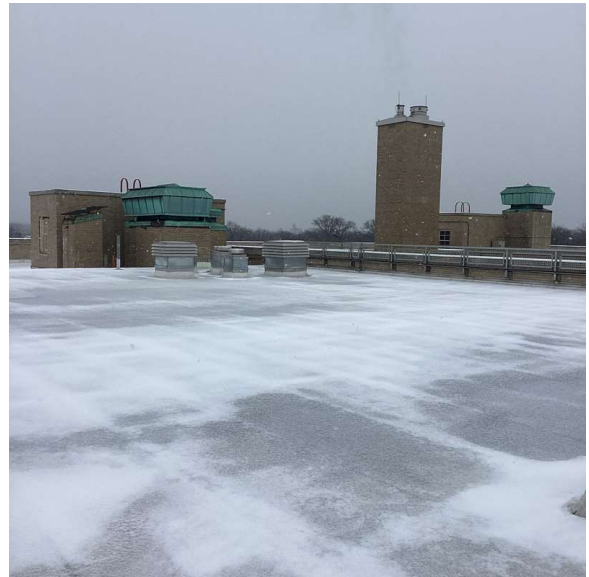
Roof 2 - North View
