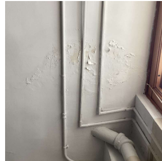
Roof 1 - Room 309 (Roof 1 - Rooms 312, 332, Roof 2 - Room 342)
