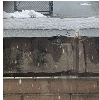
Roof 3 - Facade E
